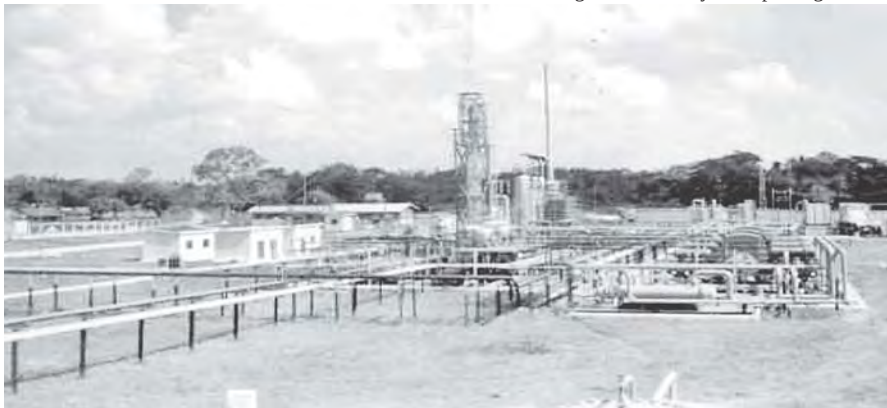
Photo shows Nyaungdon Lequified Petroleum Gas Plant.
