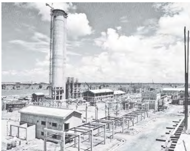
No. 4 Fertilizer Plant (Myaungdaga) construction project in progress.
