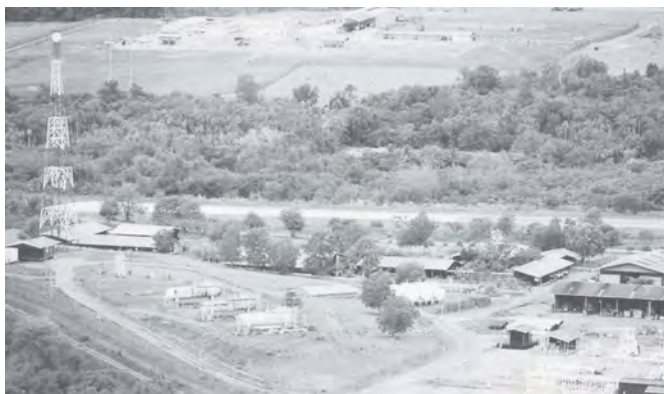
Photo shows Kanbauk natural gas pipeline centre.
