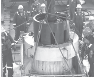
Workers onboard the Transocean Discoverer Inspiration retrieve the flange overshot tool used to remove the flange from the Deepwater Horizon BOP, on 11 July, 2010 in the Gulf of Mexico.—XINHUA
