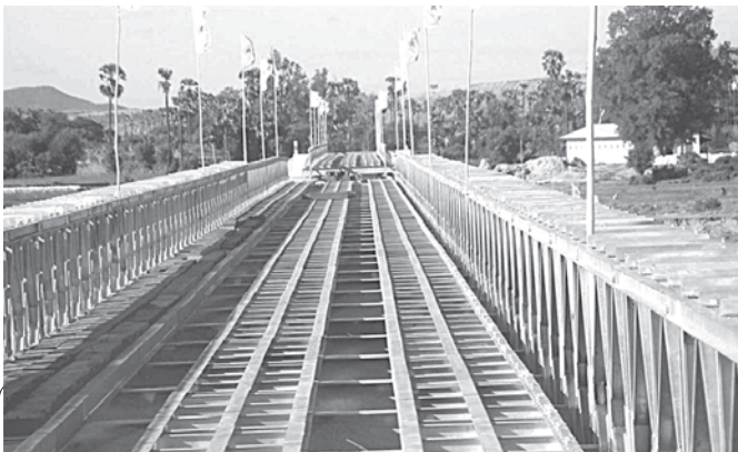
Myaukyamachaung Bridge Project on Patheingyi Road between Salingyi Township and Yinmabin Township.—MNA
