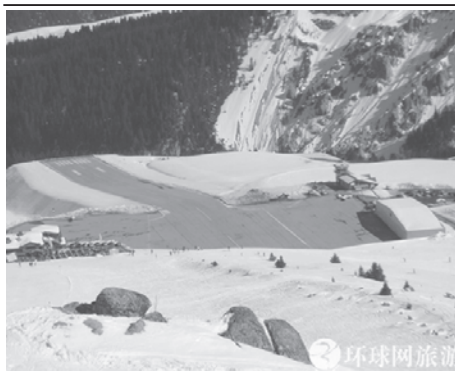
Courchevel Airport is a French airport that serves Courchevel, a ski area. The airport has a very short runway of only 525 metres with gradient of 18.5 %. There is no go-around procedure in this airport.
