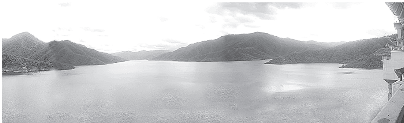
Photo shows the dam of Yeywa Hydropower Plant Project.—MNA
