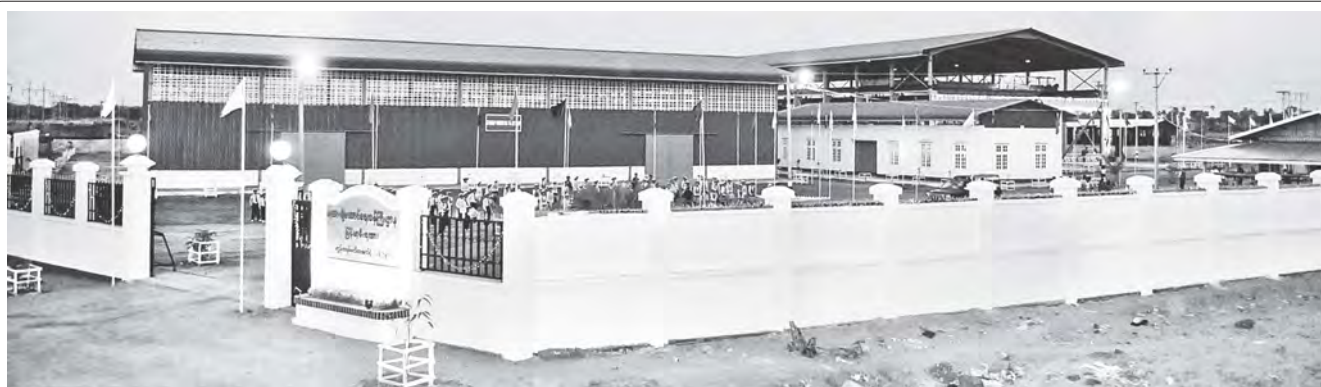
Photo shows Concrete Sleeper Factory (Pakokku) that produces 600 sleepers a day and about 200,000 sleepers per year.
