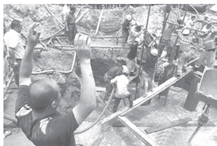
Rescuers work at a construction site in Nantong, east China's Jiangsu Province, on 8 July, 2010. A seven-year-old boy fell into a 15-metre-deep and 30-centimetre-in-diameter pile hole at the site around 6:00 pm local time Wednesday, and was successfully extricated after 20 hours' effort.
