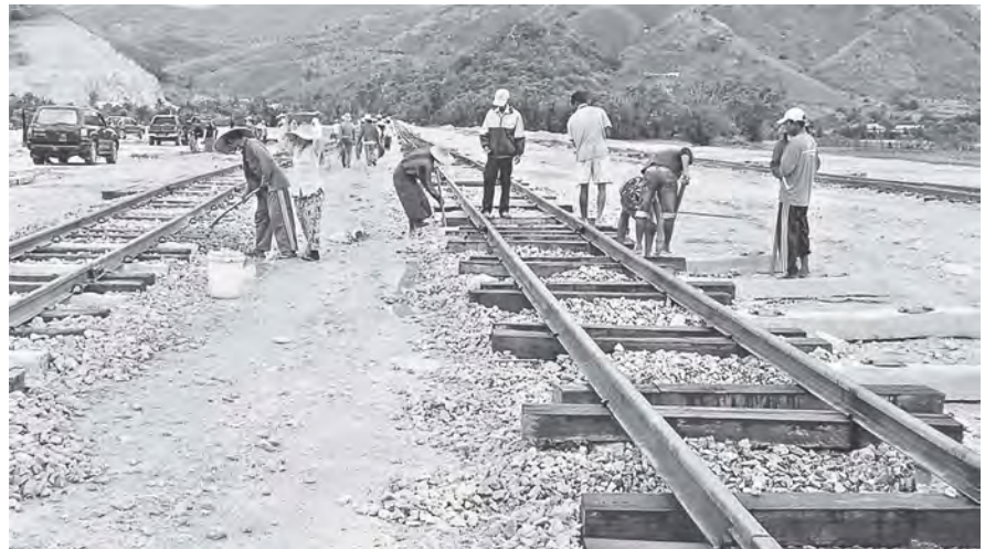
Mongnai-Kengtung railroad under construction to link Shan State (East) and Shan State (South).
