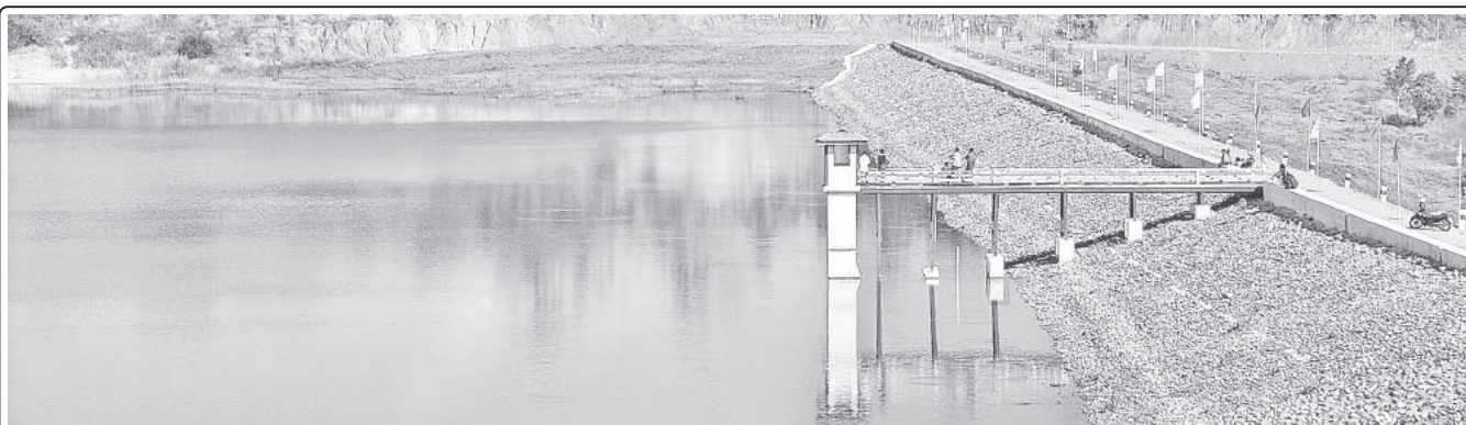
ThanUchauk Dam in Kyaukhtu Township, Gangaw District, Magway District.
