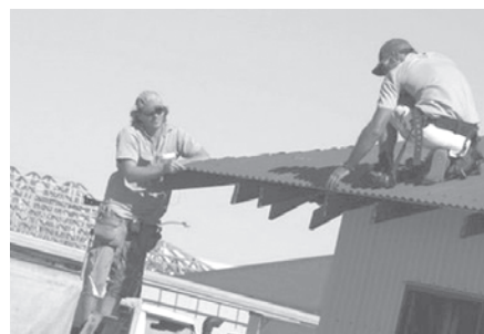
Tradesmen erect a roof on a new house in the mining town of Karratha in the north of Western Australia. New data on unemployment in Australia, seen as renewed proof of the country's resilience in the face of global economic turmoil, has pushed the dollar higher.—INTERNET
