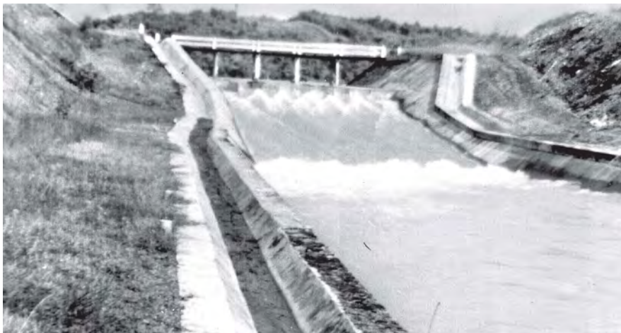
Khawa Dam releases water through spillway.
