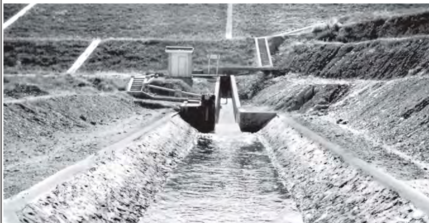
Photo shows the conduit of Khawa Dam which is a reliable irrigation facility for residents of Bago Division (West).
