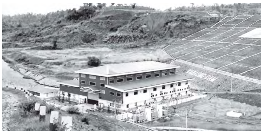
Khabaung Hydropower Plant (30 megawatts) seen with the embankment of Khabaung Dam in the background in Ottwin Township.
