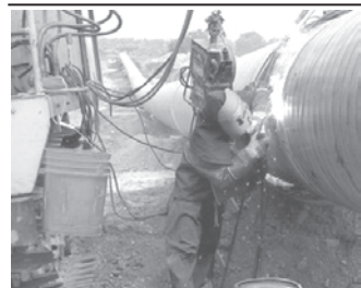
Engineers weld carbon steel pipes for India's Reliance Industries close to Hyderabad. India's billionaire Ambani brothers, who own the many arms of the Reliance Industries empire, have been signing deals and drawing up expansion plans after calling a halt to their very public five-year battle over the spoils of their father's vast business.
