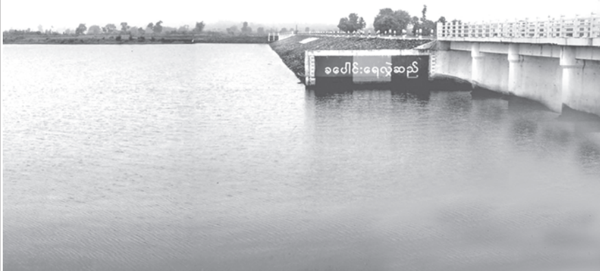
Photo taken on 25 June shows storage of water at Khabaung Diversion Weir located near Shwelaung Village of Ottwin Township.
