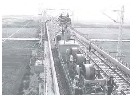
Rail workers step up installing the electric leads of the contact line on the construction site of the Baotou-Xi'an Railway, in Pucheng County, northwest China's Shannxi Province, on 27 June, 2010.
