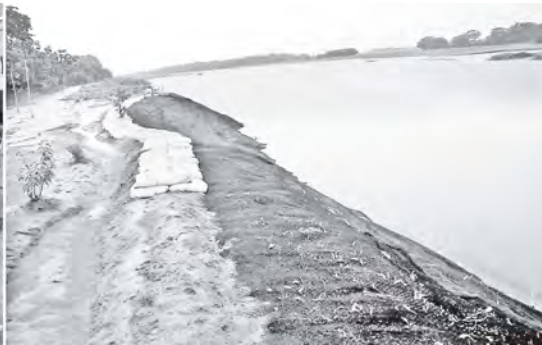
Prime Minister U Thein Sein views installation of GEO TUBE and construction of embankment for prevention against bank erosion of Ayeyawady River.
