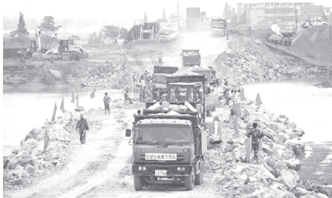
Soldiers work at the breach site of the dike at the Changkai section of the Fuhe River, in Fuzhou City, east China's Jiangxi Province, on 27 June, 2010. More than 400 workers and soldiers narrowed a 400-metre gap in the dike by more than 200 metres as of 10 pm Saturday, as floods that have killed 235 people ravaged the south of the country for the 12 th day. It is expected that the breach of the dike be repaired by Sunday night or Monday morning.—XINHUA
