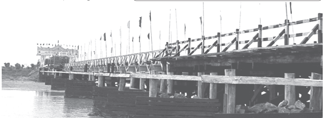
Yin Creek Bridge on Taungdwingyi-Myothit-Natmauk Road in Natmauk Township, Magway District, Magway Division. —CONSTRUCTION
