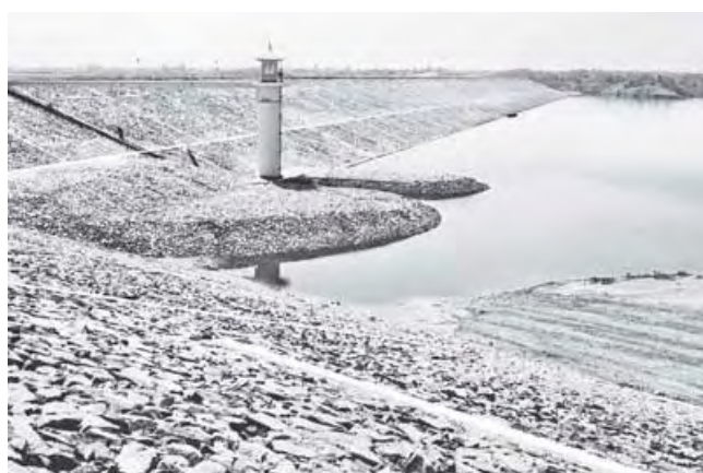
Wagadok Dam stores water.
