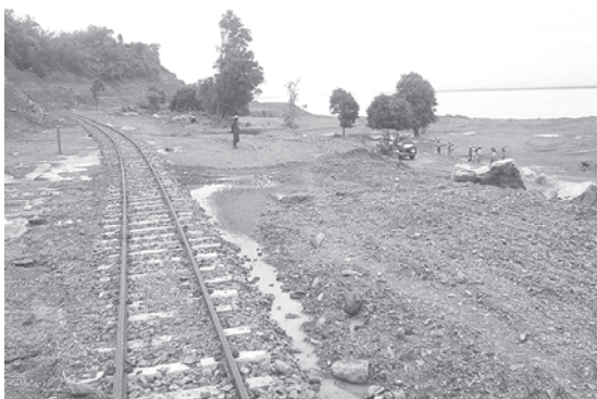
Prime Minister U Thein Sein views maintenance of railroad between Ponnagyun and Yoetayoke stations.—MNA
