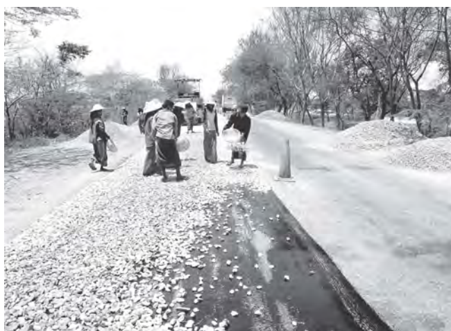
Mandalay-Meiktila highway section is being upgraded.
