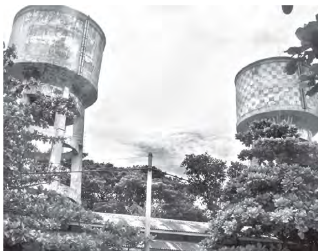
Two concrete tanks, the sources of potable water for residents of Yamethin.
