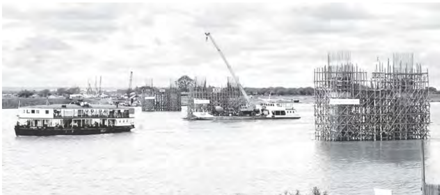
Construction site of Ayeyawady Bridge (Pakokku), the longest bridge in Myanmar.
