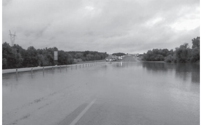
Photo taken on 14 June, 2010 shows the flooded highway connecting Stillwater and Oklahoma City in the United States. The US state of Oklahoma is under a state of emergency spread across 59 counties after severe thunderstorms ripped through central Oklahoma on Monday triggering massive flooding.—XINHUA
