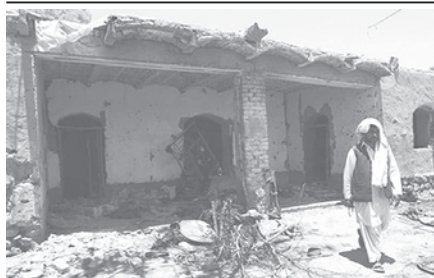
An Afghan walks in front of a house damaged in a blast during a wedding in Kandahar's Argandab district on 10 June, 2010. Scores were killed when a blast ripped through a wedding party in Kandahar province's Argandab district late Wednesday, killing 40 people and wounding dozens more, officials said. Afghan Interior Ministry spokesman said the explosion was a suicide attack.
