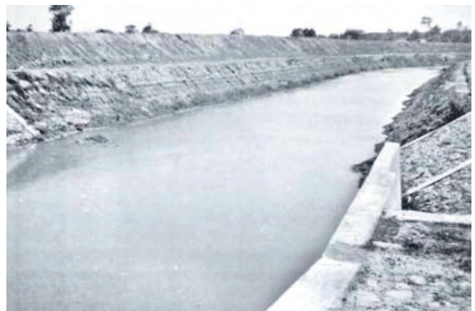
Main canal of Yenwe Diversion Weir supplying water to arable lands.
