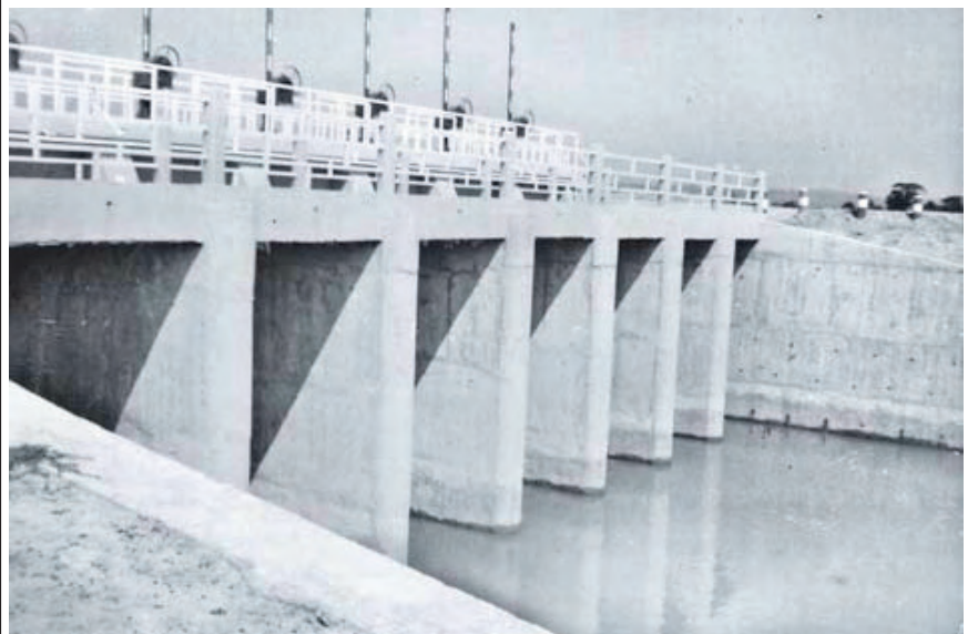
Photo shows the front view of Yenwe Diversion Weir.
