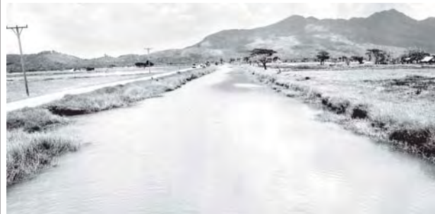
Irrigation water from Kadaik Dam distributed through canal.
