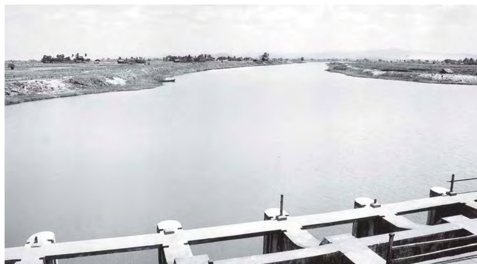
Yin Nyein Sluice Gate in Yin Nyein Creek.
