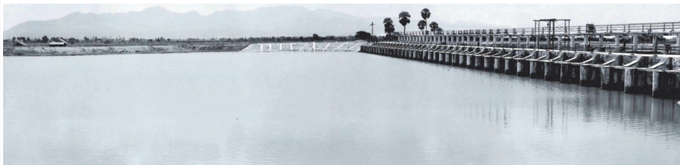
Yin Nyein Sluice Gate has been built by damming up Yin Nyein Creek near kyonehtaw Village, Paung Township, Mon State.
