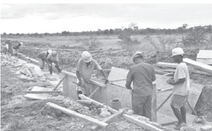
Tanzanian builders work at the site of a China aid agricultural demonstration centre in Morogoro, some 240 kilometres from Dar es Salaam, Tanzania, on 4 June, 2010.—XINHUA
