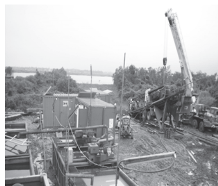
HDD (Horizontal Directional Drilling Machine) in operation to drill river floor.
