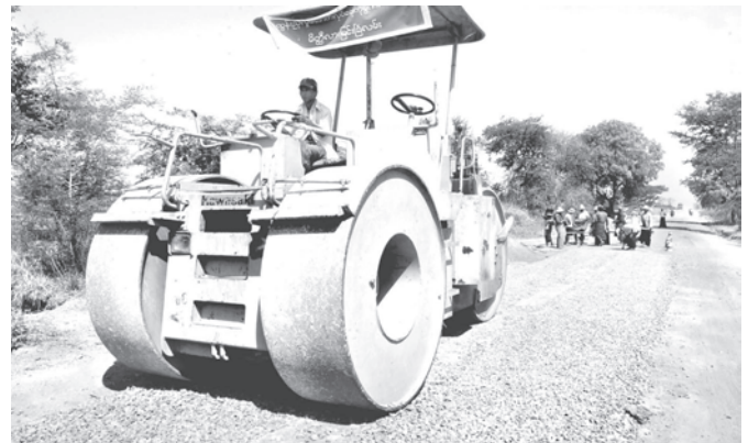
Upgrading of road with the use of machinery.
