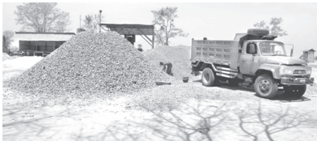
Gravels being piled at a site on Meiktila-Myingyan road section.
