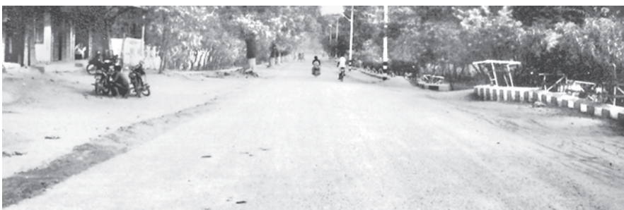
An upgraded road near mile-post 22/3 in Mahlaing Township on Meiktila-Myingyan section.
