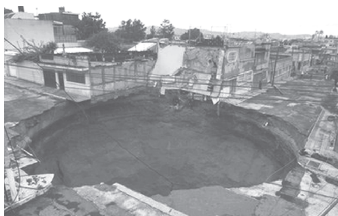
A sinkhole created by tropical storm Agatha covers a street intersection in downtown of Guatemala City on 30 May, 2010. Torrential rains brought by the first tropical storm of the 2010 season pounded Central America and southern Mexico, triggering deadly landslides.
