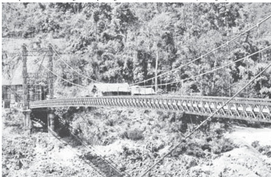
A creek-spanning suspension bridge on Myitkyina-Chipwe Road.
