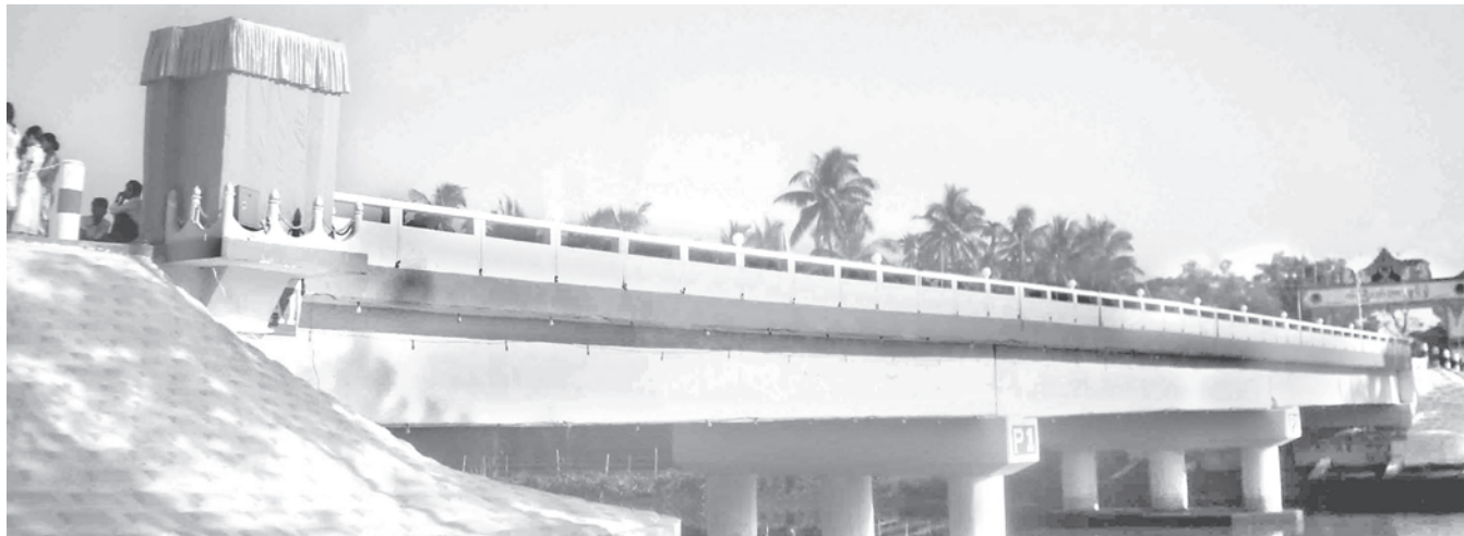
Kangyi Bridge in Ayeyawady Division that contributes to smooth and swift commodity flow.
