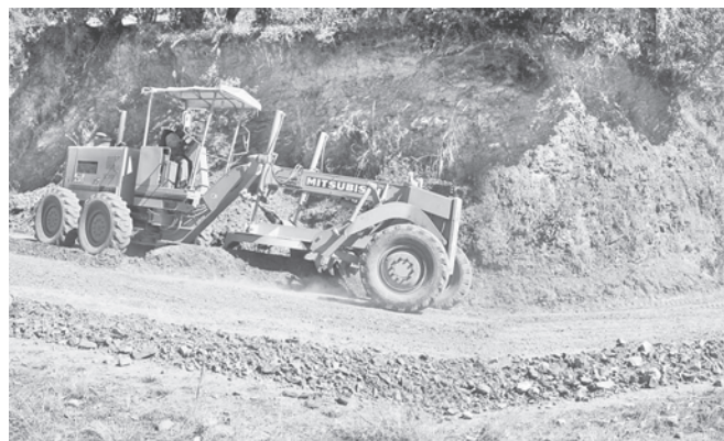
A road section in Tiddim Township, Chin State, is upgraded to a fine transport facility.
