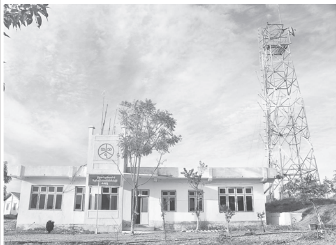
The Myanma Posts and Telecommunications has established a tower and post office each in the townships in border areas.
