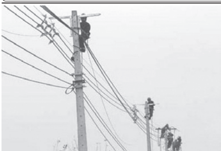
Workers repair electricity pylons and wires damaged during an earthquake in February, in a rural area near Santiago on 26 May, 2010. The 8.8-magnitude earthquake on 27 February was one of the world’s most powerful in a century and killed more than 700 people.
