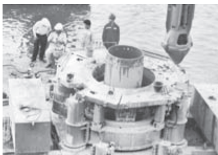
Bore piling at the rocky ground.
