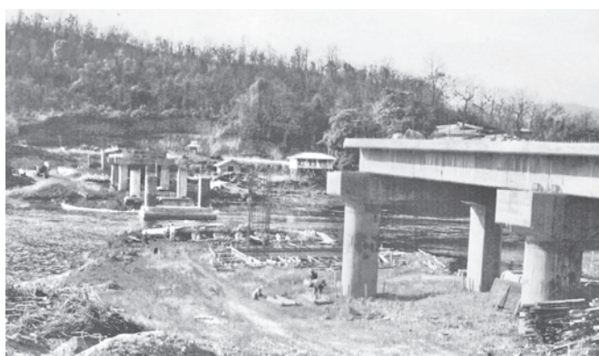
Construction of Dokhtawady Bridge (Hsipaw) seen on 9 May.
