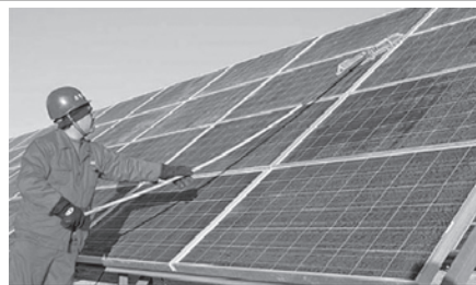
An employee cleans solar panels at a power plant in Dunhuang, Gansu province.—INTERNET
