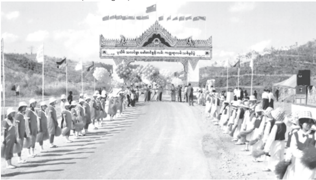
The opening of Pathein-Thalatkhoa-Mawtinsun Road in progress.
