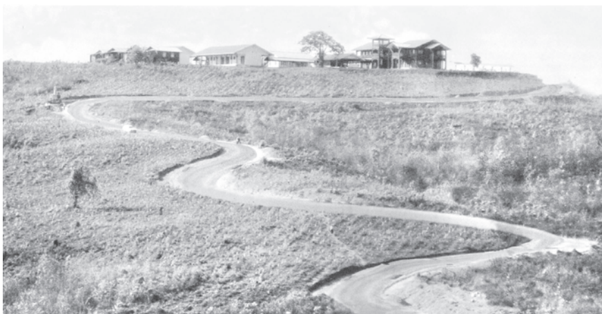
A road section of Pathein-Thalatkhoa-Mawtinsun Road, which was commissioned on 14 May.
