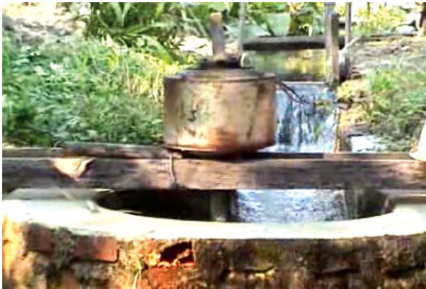
Small hydroelectric generator in a village
