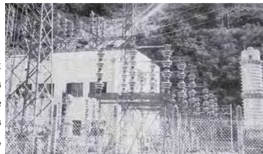
Centrale hydro-électrique de Lawpita (Photo: Karenni Development Research Group)
