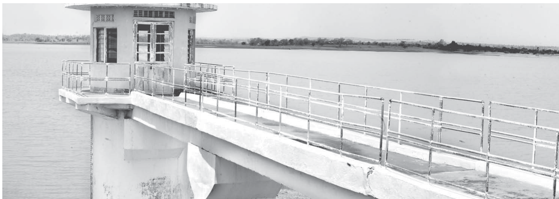
Photo shows Chaungkauk dam in Meiktila Township.
