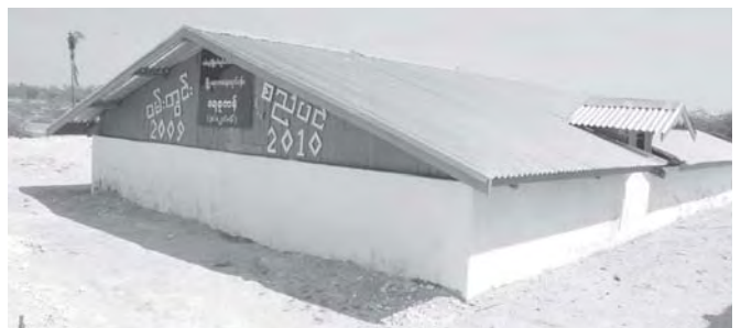
Water pumping station in Wundwin.
