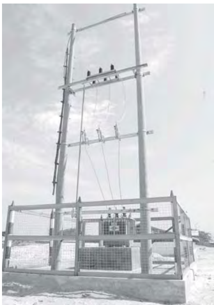
A transformer to operate water pump for supplying water.
