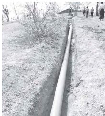
Water pipelines being laid onto Thein Hill.
