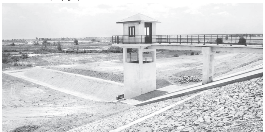
Control tower and conduit of Yeboke Dam Project being implemented in Hlaingbwe of Kayin State.
