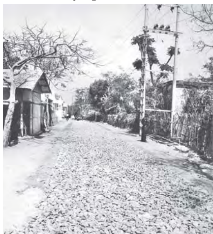
Paving of a road in Myaing Township.
