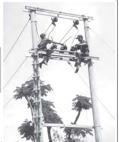
Workers connecting 11-KV power lines from Kanma natural gas power plant for power supply. (Byline on page 7)
