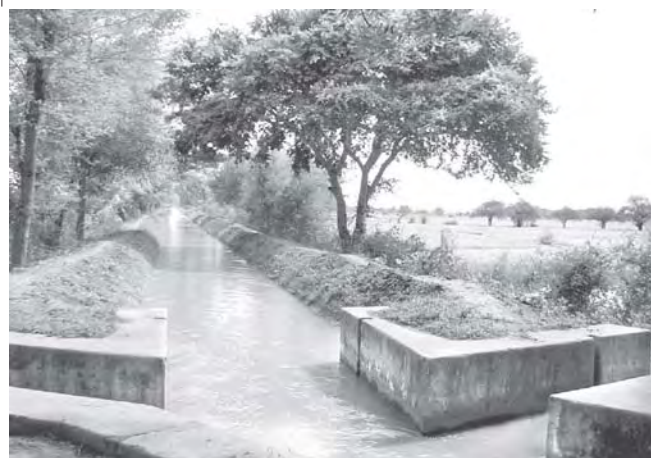
Letpanchepaw water pumping station.
