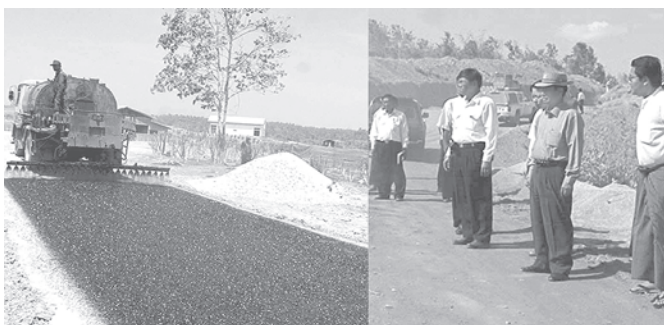
Minister U Khin Maung Myint looks into construction of Pathein-Thalakkhwa-Mawtinsoon Road.
