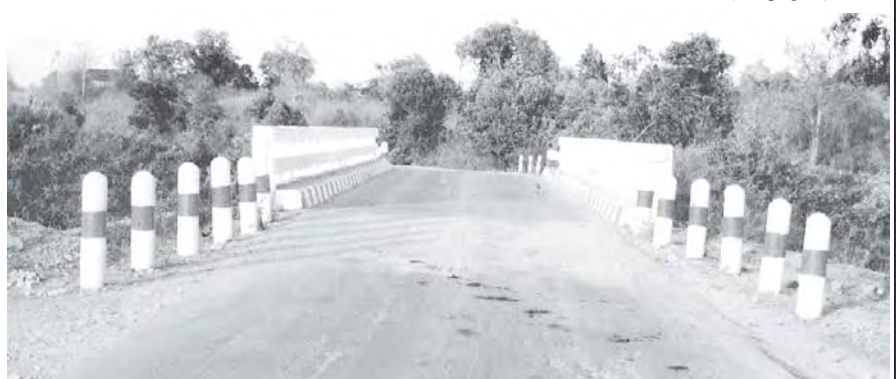
A bridge on Pathein-Thalakkhwa-Mawtinsoo Road.
