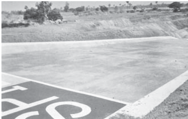
Spillway of Kandaunt Dam.
