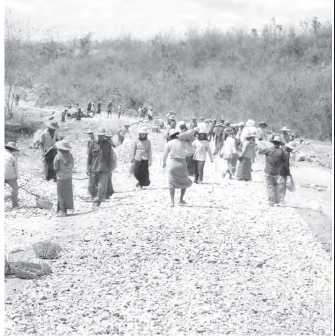
Workers at Pathein-Thalakkhwa-Mawtinsoo Road.
