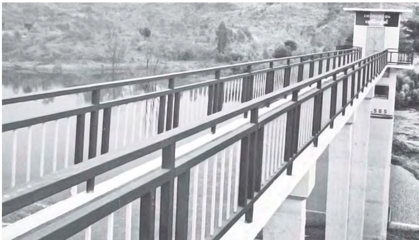
Control Tower of Bawditahtaung Dam.
