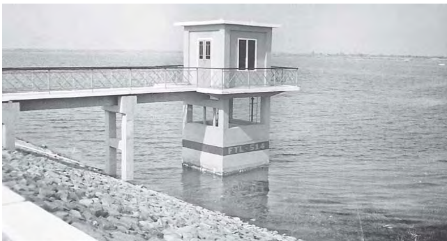
Water control tower seen at Linpan Dam.
