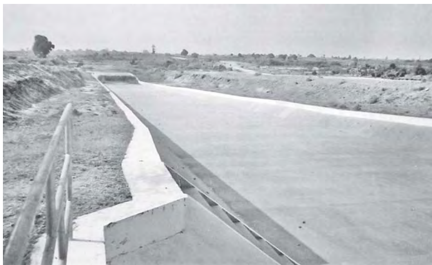
Photo shows spillway of Linpan Dam.
