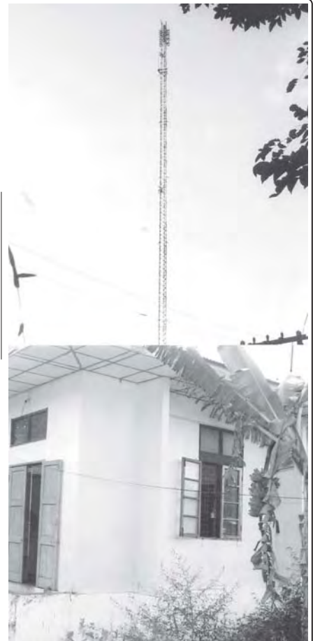
TV Re-transmission Station established in Minhla.
