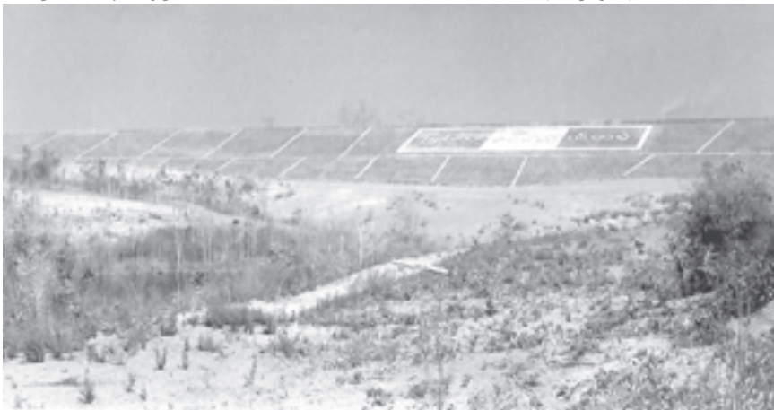
Myittha Dam, located near Pyintha Village of Gangaw Township, will irrigate 12,000 acres of lands.
