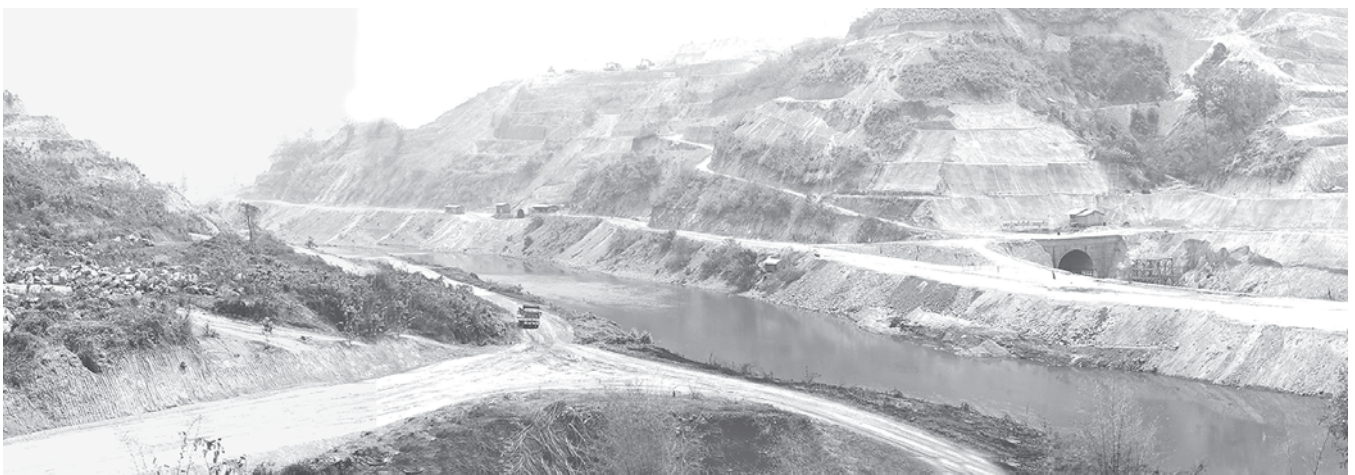
Photo shows Thaukyaykhat (2) Hydropower Project.—MNA
