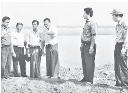
Officials explaining construction of retaining wall.
