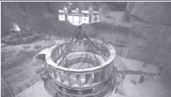
Workers proceed with hoisting installation of the socket ring with a diameter of 14.38 m and weight of 362 tons for the gigantic hydropower unit set with a single unit capacity of 800,000 kilowatts, at the Xiangjiaba Hydropower Station of Yibin City, southwest China's Sichuan Province, on 23 March, 2010.—XINHUA
