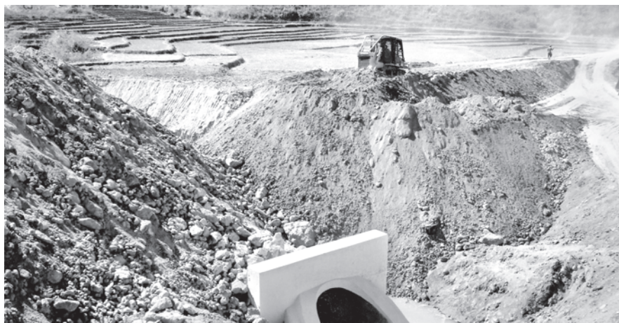
Ten-foot-tunnel-type bridge at Kengtung-Yanlu road section.
