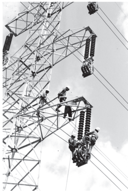
Workers of Ministry of Electric Power No. 2 installing power lines.
