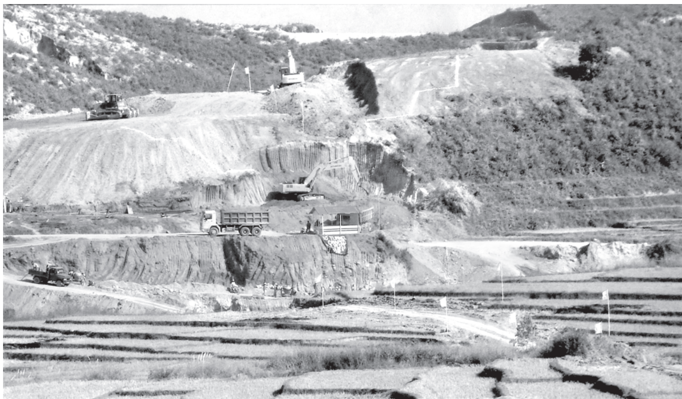
Ministry of Rail Transportation constructing Kengtung-Yanglu railroad section with the use of heavy machinery for better transport of local people.
