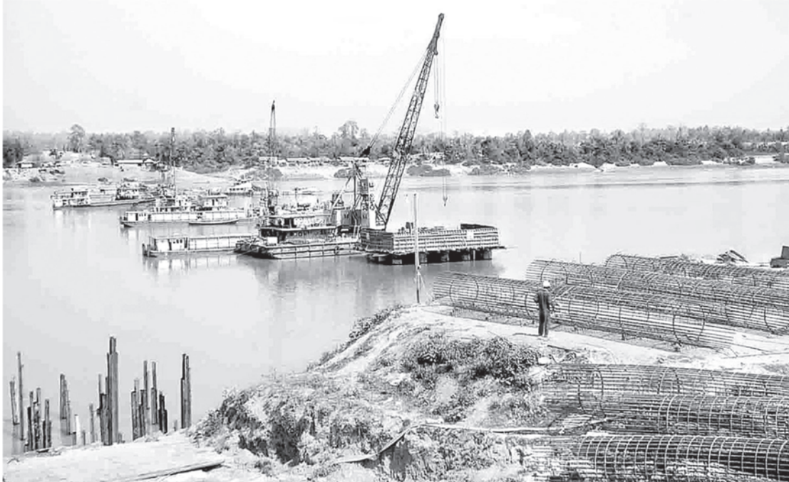
Rail-cum-road Ayeyawady Bridge (Sinkhan) under construction.
