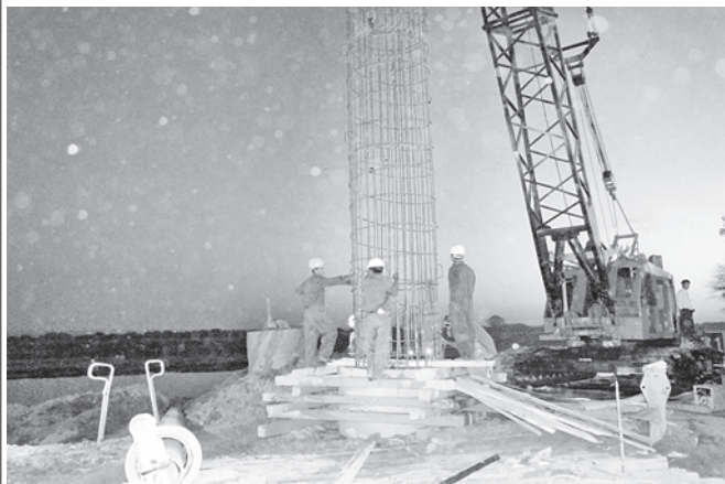
Ayeyawady Bridge (Pakokku) construction on Pakokku bank.
