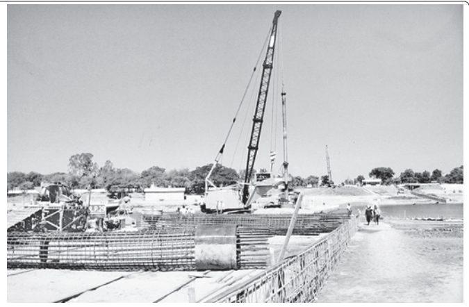
Construction being carried out by heavy machinery.
