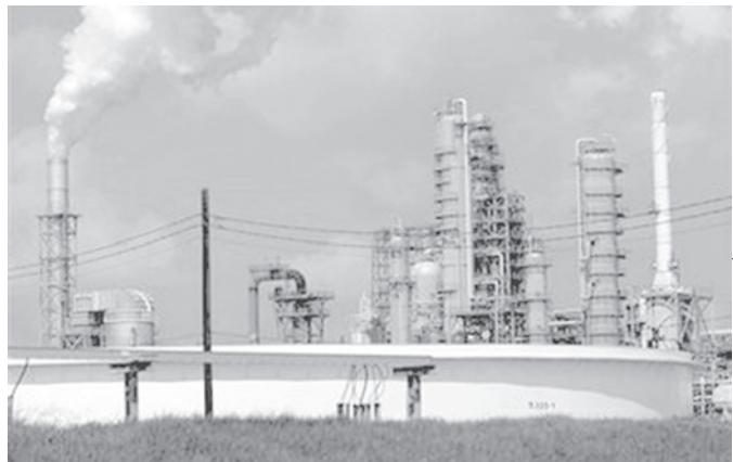
File photo shows The Valero St Charles oil refinery is seen during a tour of the refinery in Norco, Louisiana on 15 August, 2008.
