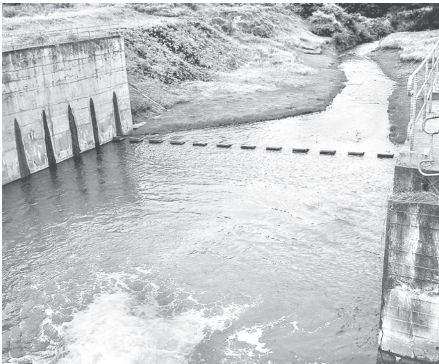
Kinmuntaung Dam irrigates paddy fields with an over-six-mile channel.
